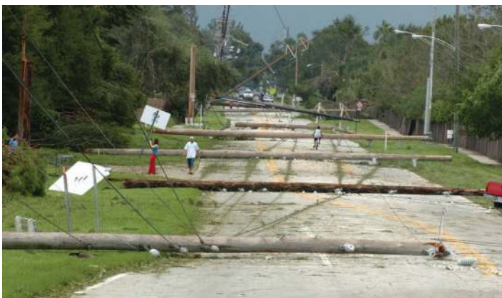
Wind damage from Hurricane Charley, August 2004, Orlando, FL/Orlando Sentinel, copyright 2004
