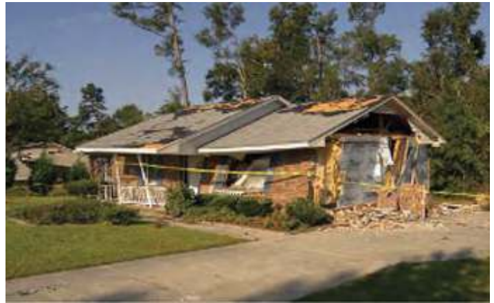
Hurricane Frances tornado damage, Sumter County, SC, September 2004/Marvin Mauman, FEMA
